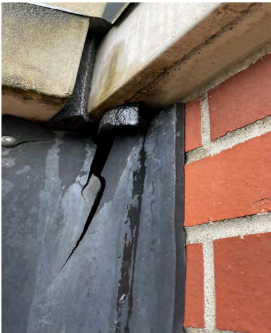
Pedestrian Bridge Failed Flashing and Seal
