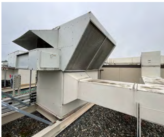
DX/HW VAV Rooftop Unit
