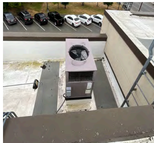
Packaged Heat Pump Rooftop Unit
