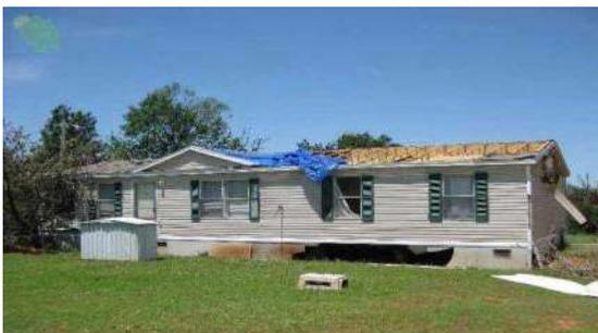
Although much of the roof is missing, the structural ribbing of the roof system is still intact.
