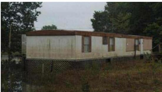
Visible water line above the floor system.
