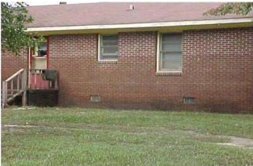
The visible water line on the residence is higher than 18 inches on the first floor.
