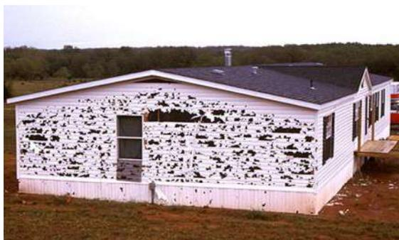
Nonstructural components of one wall have sustained damage.
