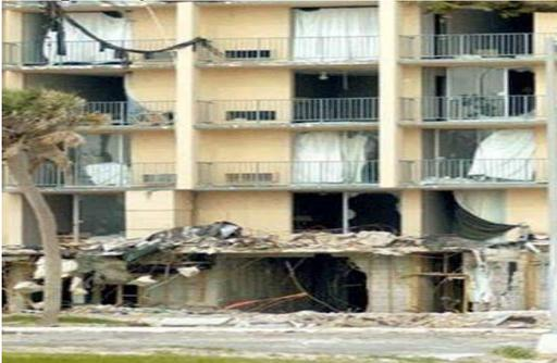
Based on this view, at least 12 units should be classified as having major damage. All units in an apartment building will not necessarily have the same damage level.
