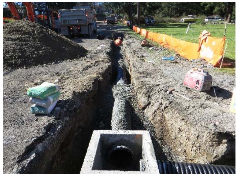
New storm sewer drain pipe and catch basins have been installed to capture storm water runoff. The storm system will include a pretreatment catch basin and underground detention vault.
